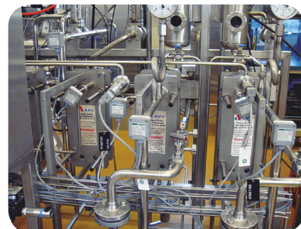
Sensors in crowded places are a challenge, particularly where impulse line length must be kept at a minimum for cleaning. Source: Baumer
